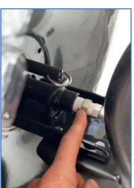
Install hose reel on to hose cart yoke. Tighten bolts.
